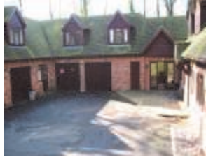
High Tech Offices
